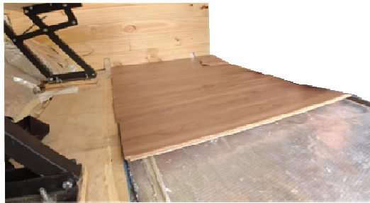
Thermal Insulation on the floor, and real wood can be installed
